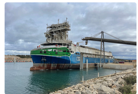
Trans-shipment vessel at the T-Port at Lucky Bay, South Australia
